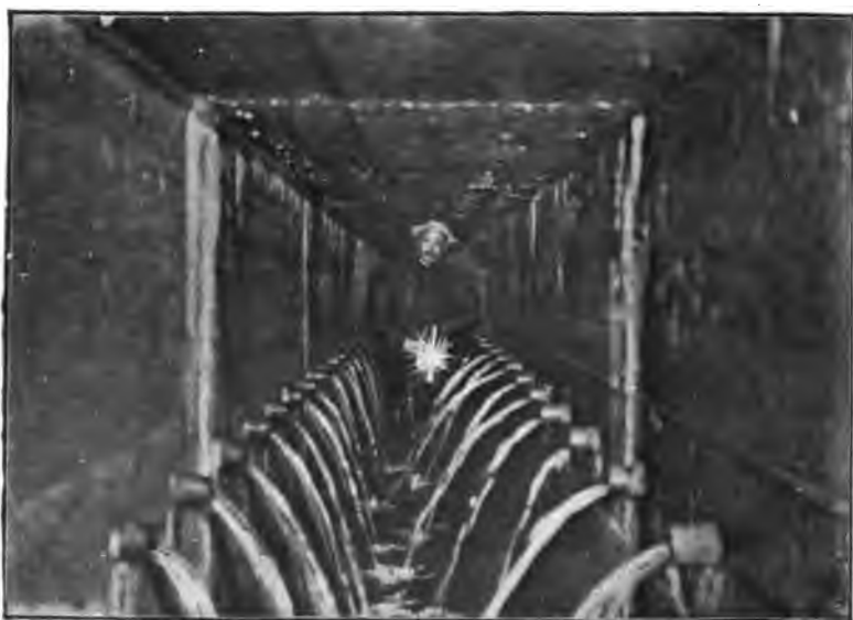
FIG. 14.—Subterranean Water Tunnel and Feed-wells: California.
